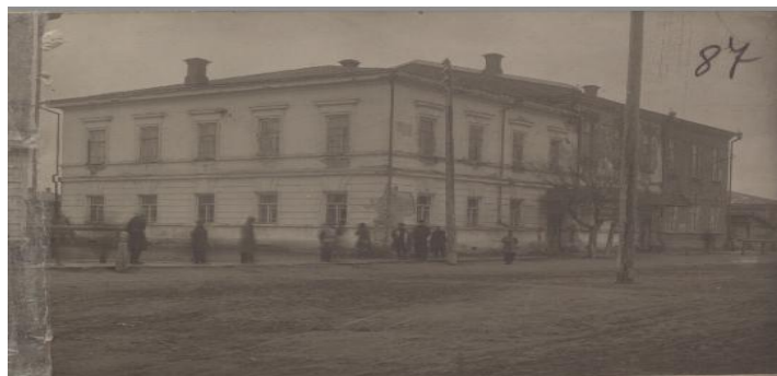
Figure 1. Building No. 60. Building of Kazakh pedagogical college, 1926 [12; 87].
