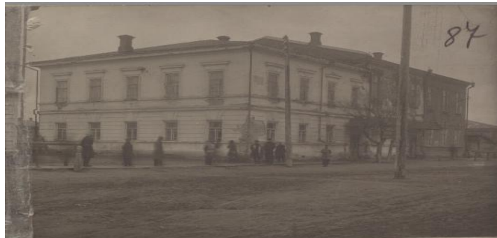
Figure 1. Building No. 60. Building of Kazakh pedagogical college, 1926 [12; 87].
